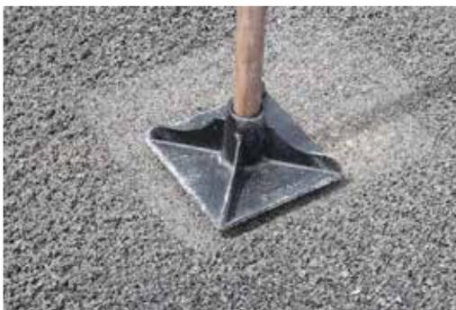
It may be necessary to compact the native soil/subgrade prior to base construction.
